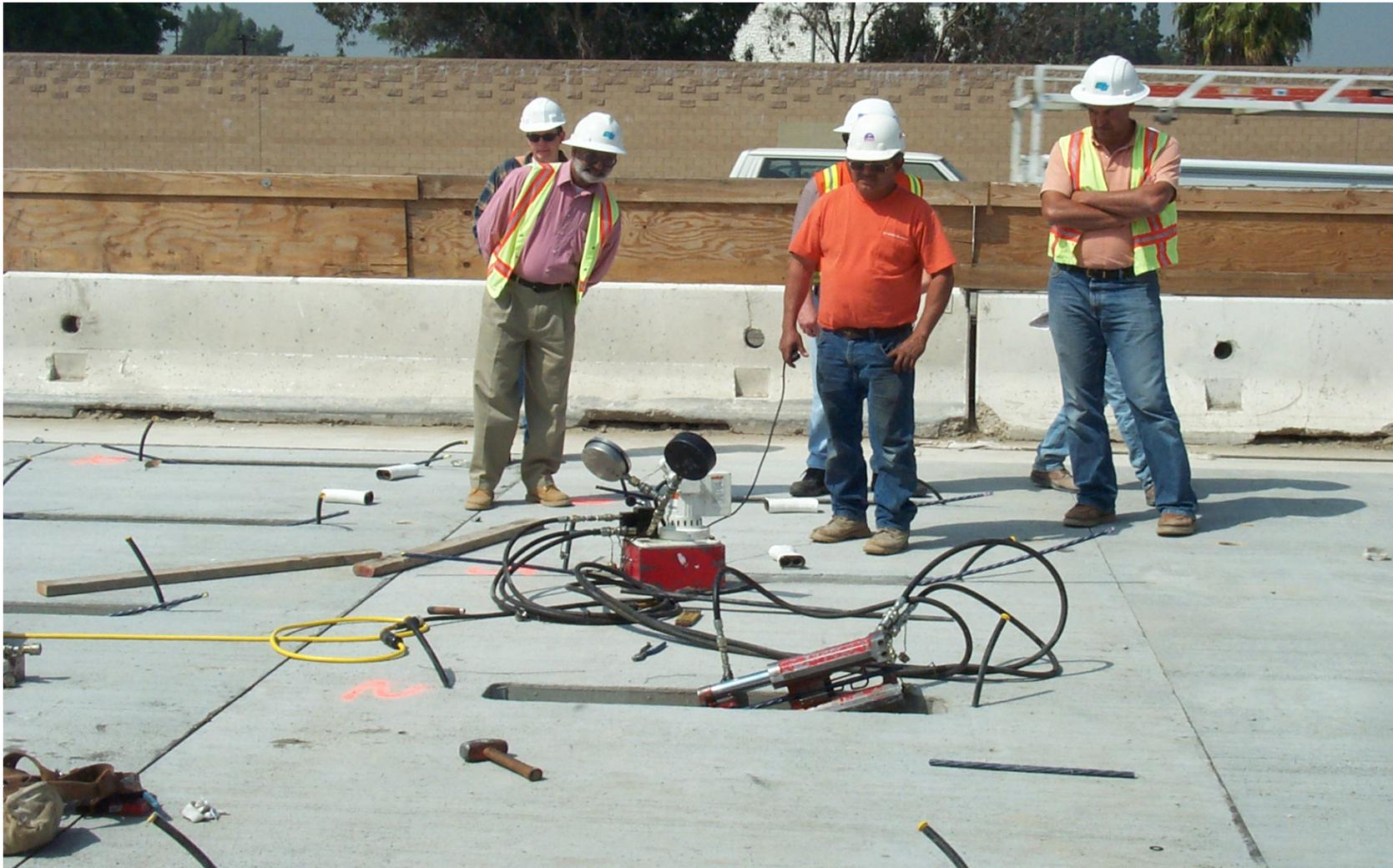
Epoxy Coated PC strand being tensioned for one directions of the PC pavement sections
