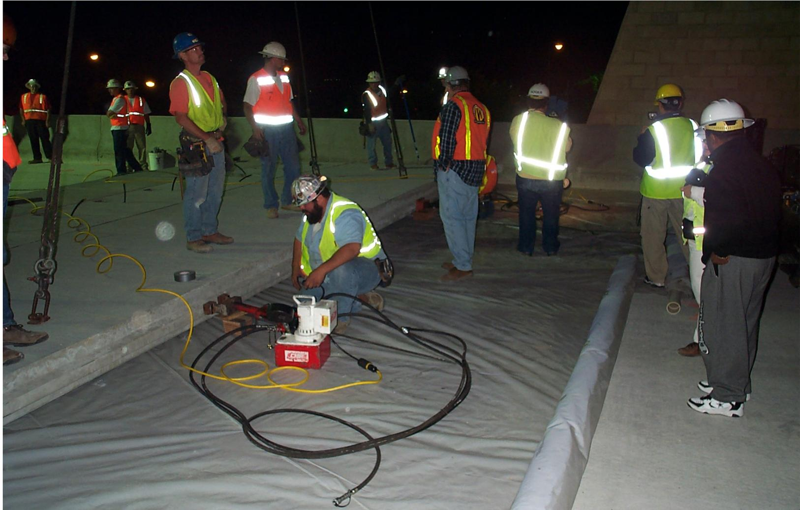
Epoxy Coated Strand was used for the Post Tensioning of the slabs
